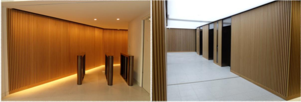
38mm deep Dalhem ribs were specified for 1 King William Street to visually offset the 20mm gaps which in turn were chosen to give excellent acoustic control at 35% open area. Dalhem Ribba is available in the UK only through LSA Projects Ltd.
