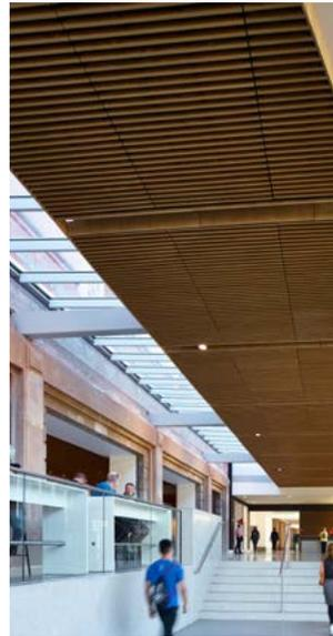
All panels in stock are available in wall and ceiling format and in either 1800mm or 1200mm x 600mm. All pieces are in style 7-501 as section drawing; with 20mm (w) x 45mm (d) blades and 40mm spaces.
